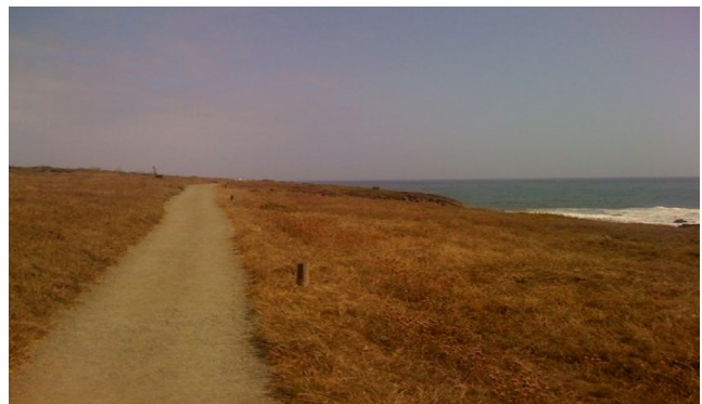
This segment of the old Fiscalini Ranch Marine Terrace Trail (i.e., Coastal Trail) has an unimproved earthen surface of approximately 4 feet in width and supports moderate to high levels of multiple use.
