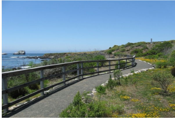
This “Improved Natural Surface” segment of the Coastal Trail immediately adjacent to Highway 1 and a public access parking lot in San Luis Obispo County includes road base, trail tread, fencing to restrict bluff access and a rock border to further guide control access.
