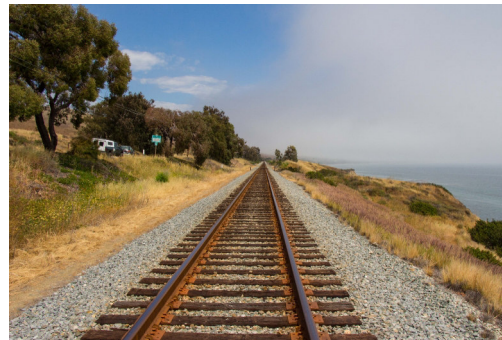
US 101 and UPRR run parallel for approximately seven miles west of Refugio State Beach, often at or near the bluff edge, which limits space for development of a bluff top Coastal Trail. Caltrans has indicated a willingness for siting segments of the Gaviota Coastal Trail within the ROW.
