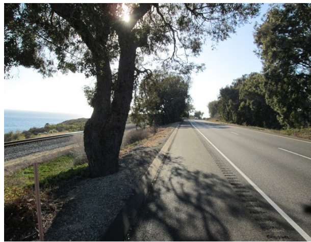
The US 101 road shoulder trail of the western Gaviota Coastal Trail segment would utilize Caltrans ROW outside the edge of the road shoulder. This would require installation of protective concrete K-rail barriers between highway travel lanes and the trail, retaining walls in some areas, tree removal and often a fence to separate the bike path from the UPRR.
