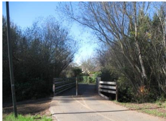
County trails employ large free span bridges to cross major streams. The Obern Trail in Goleta has 5 free span bridges of 25-70 feet long that cross Atascadero and Maria Yganica Creeks, both designated Environmentally Sensitive Habitats that support riparian woodlands and sensitive species (e.g., steelhead trout, western pond turtle).
