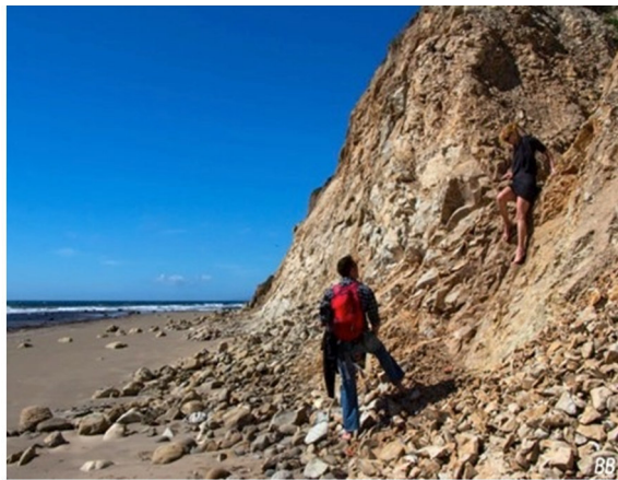
The existing beach access trail descends a small draw or canyon with the last 6-7 feet a relatively steep descent. Improvements to this access trail could include use of railroad ties or wooden stairs, with the lower 10-15 feet constructed on wooden pilings.
