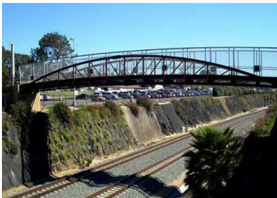
Completion of the Gaviota Trail would require construction of two new bridges across the UPRR, as preferred by the CPUC/ UPRR, similar to new bridges in Solana Beach (above). Bridges are typically prefabricated with 26 feet of track clearance; estimated cost for a new bridge at Paradiso del Maré is $1.5 million (County of Santa Barbara 2013b).
