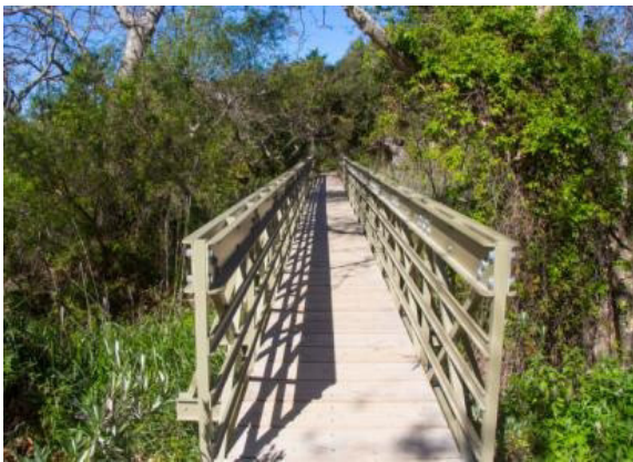
Completion of the Gaviota Coastal Trail would require construction of ten new larger creek bridges of 30 to 120 feet in length similar to this 80 foot-long bridge on El Capitan Creek. Bridges would be of metal, wood or recycled material, about 5 feet-wide and often of span construction, with foundations or abutments built outside of creek channels.
