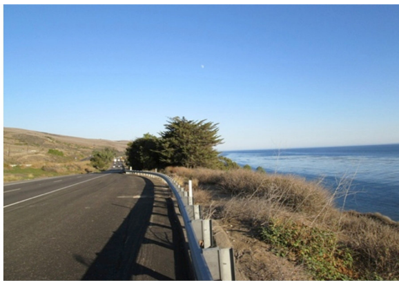
An estimated 3.5 miles of steel guard rails or concrete "k-rails" may be required to separate the US 101 road shoulder trail from high speed traffic along US 101, even with widening of the road shoulder to 10 feet.
