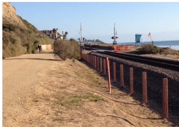
The heavily used San Clemente Coastal Trail parallels the busy Los Angeles to San Diego rail line which carries 52 daily trains; safety is provided by a low wire fence; note at-grade pedestrian rail crossing to beach (background).
