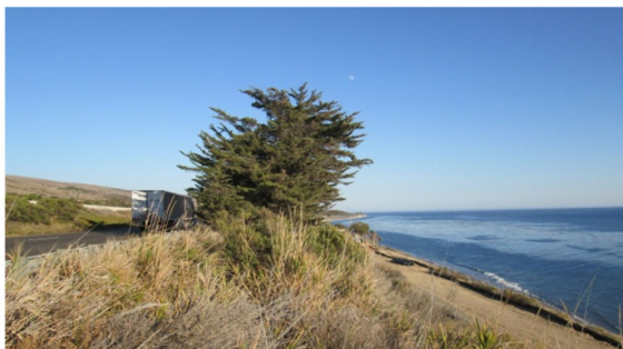
This segment would be a US 101 corridor trail for 0.9 miles from Arroyo Quemada Creek west to West of Arroyo Hondo Creek along the highway shoulder; Caltrans ROW north of the UPRR ranges from 11-14 feet to as wide as 50 feet, meeting Caltrans standards for road shoulder trails.
