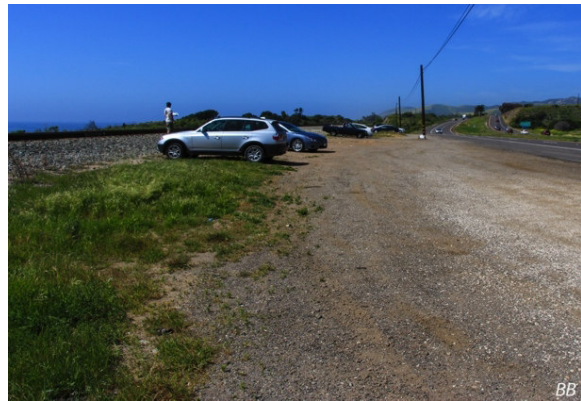
The 40-foot wide shoulder of US 101 at Canada San Onofre has a long history of providing free public parking. This shoulder is sufficiently wide to accommodate the proposed Coastal Trail segment and continued public parking between US 101 and UPRR.
