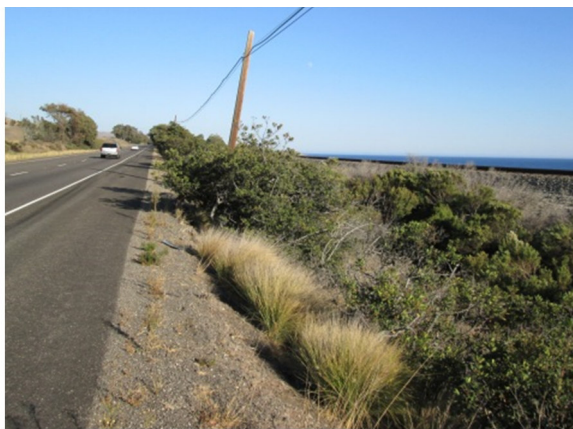
East of San Onofre Beach, US 101 ROW drops off 4-6 feet into a shallow drainage between the road shoulder and UPRR. This may require use of retaining walls and possibly relocation of utility poles along this segment.
