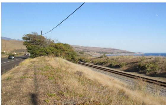
This segment of the trail would be constructed as a paved bike path within 30-40 feet of Caltrans ROW north of the UPRR; design challenges include use of protective barriers along US 101 and the UPRR, retaining walls, mature trees and utilities.
