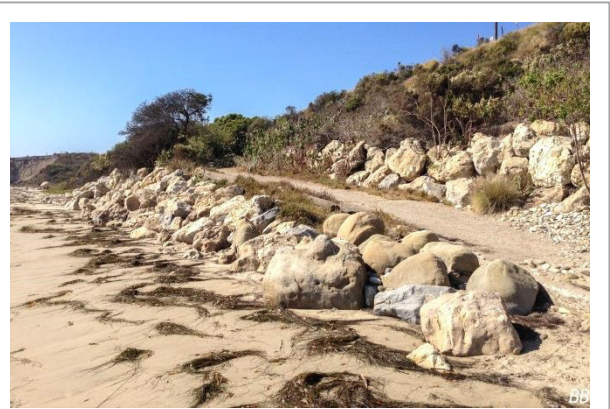
Past repairs of the Aniso Coastal Trail included installation of almost 500 feet of rock revetment to protect the trail from erosion as well as this beach access ramp. Similar improvements are needed along the currently damaged segment as the location of the UPRR precludes landward trail relocation.
