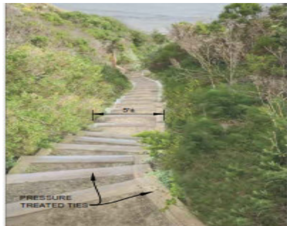
The proposed Naples beach access trail would be improved with stairway of railroad ties or other natural material in the gully bottom. A 20-25 feet-high stairway would be needed to reach the beach where this canyon falls steeply down to the sand (photo is a simulation).
