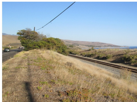
In some areas, US 101 ROW includes relatively wide open and level areas with ocean views to accommodate the Coastal Trail. These wider areas may not require retaining walls, removal of trees (background) may be required.
