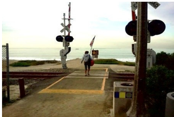
Completion of the Gaviota Trail would require three UPRR at-grade crossings similar to crossings in San Clemente (above). At-grade crossings are the least expensive crossing technique and can include pedestrian gates, warning signals and rubberized tread. While not preferred by the CPUC and UPRR, such crossings may cost $350,000 +/- to permit and construct (County of Santa Barbara 2011).
