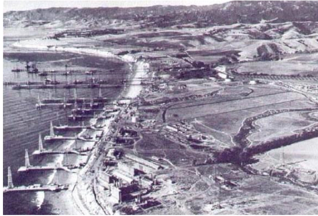
The eastern Gaviota coastline was heavily developed with oil and gas production facilities in the late 1920s and early 1930s. Remnants of oil production remain, such as degraded roads that could be reutilized for segments of the Gaviota Coastal Trail.
