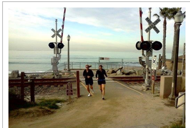
This at-grade pedestrian crossing is one of nine in four miles of the Coastal Trail in San Clemente. These at-grade crossings were installed to improve safety and reduce unsanctioned crossing. Similar public safety benefits could occur with installation of formal at-grade crossings on the Gaviota Coast.
