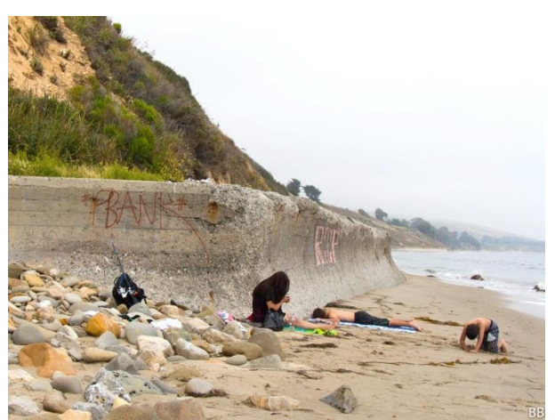
Over 1.5 miles of seawall have been constructed along the Gaviota Coast, including this 0.7-mile segment south of Arroyo Hondo. To avoid incremental armoring of other sections of Coast, the County should pursue longer-term planning, including managed retreat of UPRR and US 101 (as needed).
