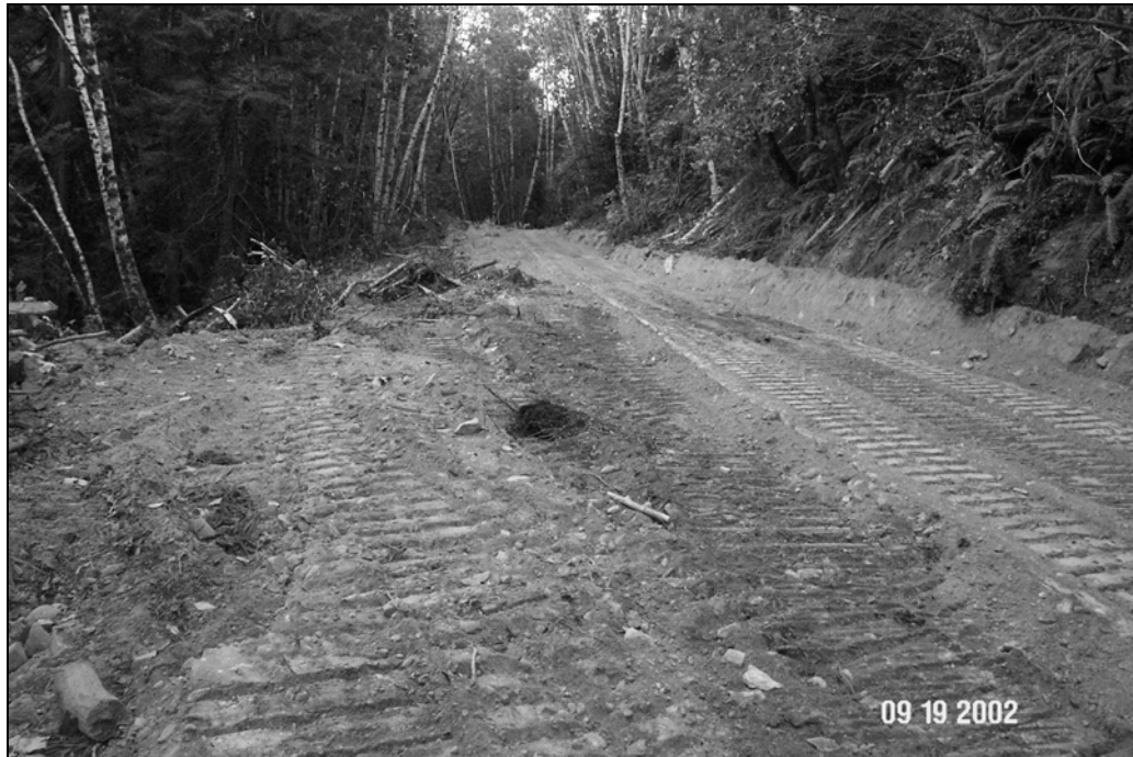
Figure X-D-26. Site # 5, 1312 Lower Road, before excavation. A potential road fill landslide was excavated at this site. Unstable outboard road fill was excavated and stockpiled locally along the cutbank behind the site, creating an outsloped road surface (see below).
