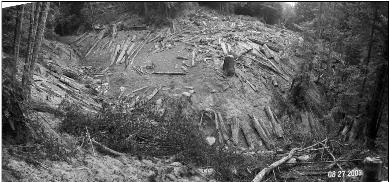
Figure X-D-19. Site # 3, 1311 Road, after excavation. This is a 2 shot panoramic compilation photo taken from near the same location as the previous picture. The site has been completely excavated, large woody debris removed from the fill during the excavation has been redistributed along the stream crossing slopes and seed & mulch has been applied to the bare slope areas.
