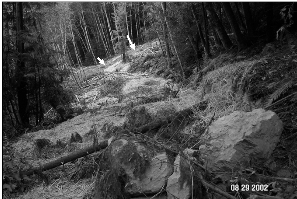
Figure X-D-17. Site #13, 1305 Road, after excavation. This picture was taken from the same viewpoint as Figure X-D-16. The unstable road fill has been completely excavated, mulched and seeded, leaving an outsloped road surface. In the background is one of the main spoil sites for this road. The sloped surface can be seen extending up above the old road bench (see arrows).
