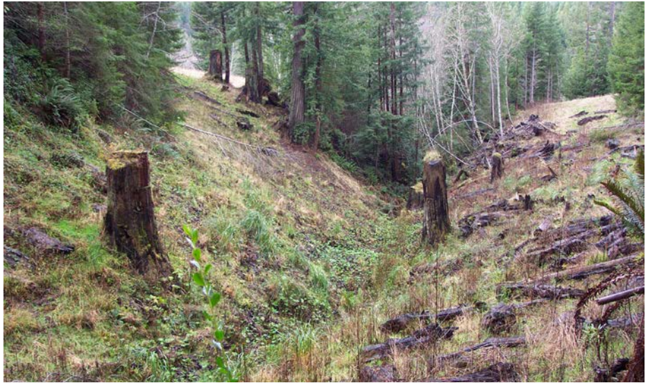
FIGURE 266D. Four years later, the site showed significant revegetation, and minimal channel adjustment (scour) or surface erosion.
