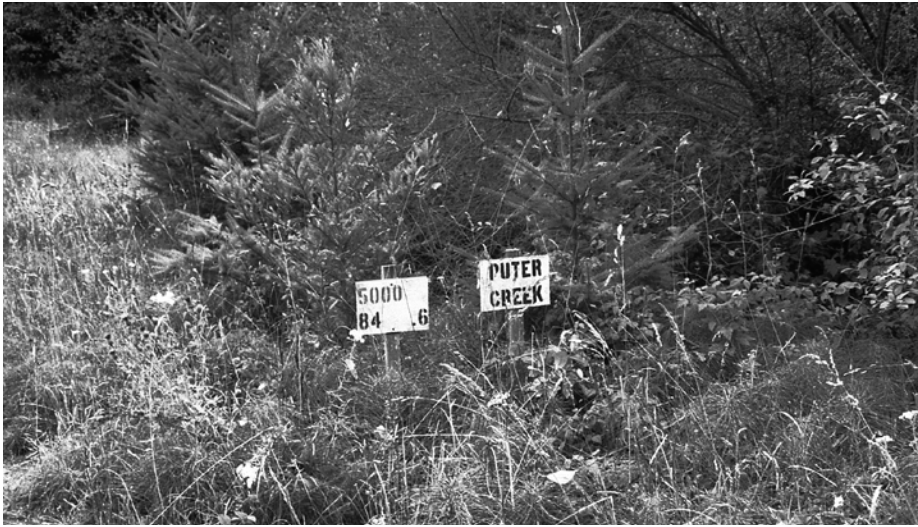
FIGURE 239. Culvert signing is an integral part of developing a culvert and drainage structure inspection and maintenance plan. Included at this crossing are the stream name (Puter Creek), the name of the road (5000 Road), the diameter of the culvert (84") and its location (0.6 miles from the beginning of the road). The signing can also be color coded (e.g., green, yellow, red) to indicate whether or not it is prone to plugging or other maintenance needs.
