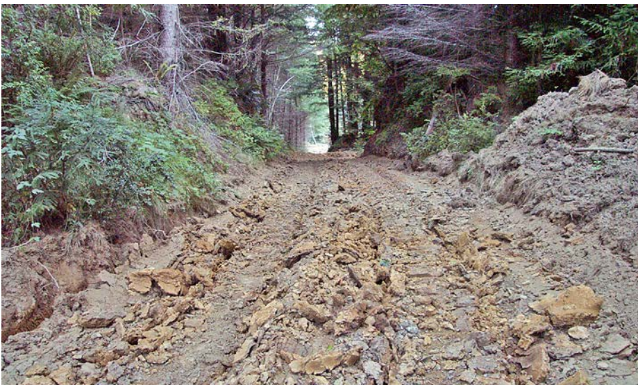
FIGURE 284B. A road after ripping and decompaction.
