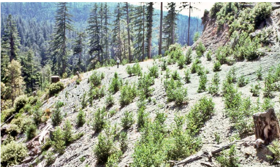
FIGURE 273B. Using Inplace Outsloping (IPOS) techniques, the rocky sidecast soils were excavated and placed against the tall cutbank of this dry ridge. Woody debris was separated from the dirt and chipped for mulch. Three years later, alder trees have invaded the bare soil surface and were rapidly growing. Minor surface erosion and rilling had occurred while the surface was sparsely vegetated, but there was no sediment delivery to a stream (note person for scale) (RNP).
