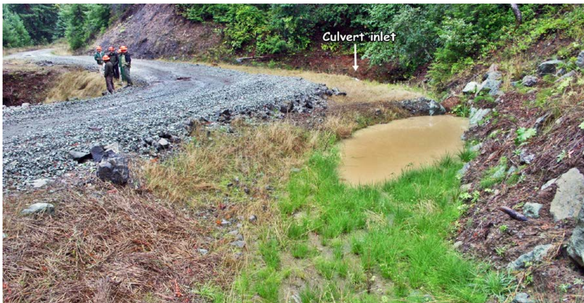
FIGURE 237. Roadbed structural deterioration caused by vehicle traffic (especially commercial traffic) on wet subgrade soils with little or no surfacing. Wet weather road use limitations (gating) or road surfacing (with base and surfacing materials) are preventive solutions to this potentially expensive maintenance problem.
