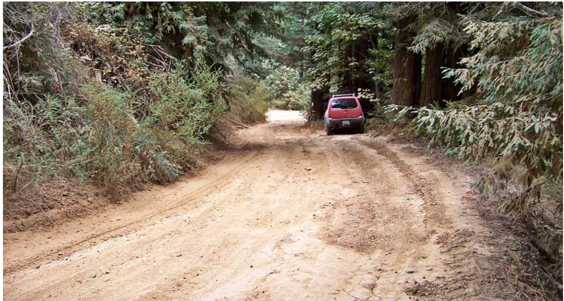
FIGURE 225A. Native surface permanent road on a rural subdivision was insloped, bermed, deeply rutted and hydrologically connected to a nearby stream prior to upgrading.
