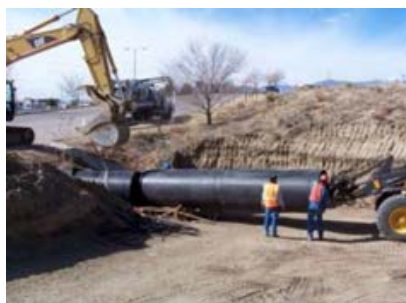
FIGURE 220. Sliplining technique for trenchless pipe installation.
