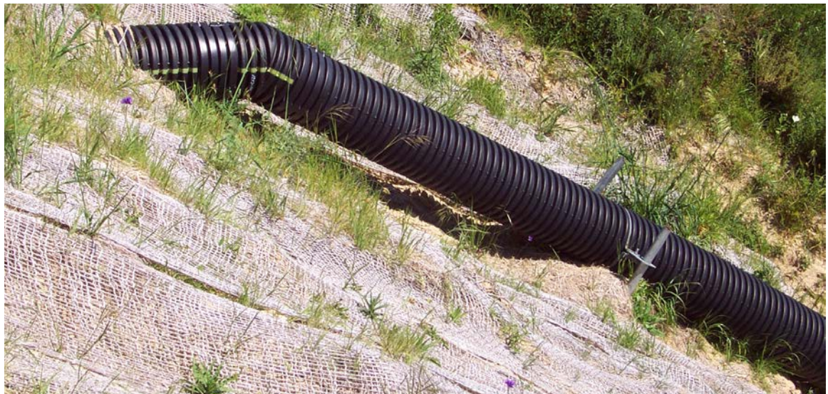
FIGURE 162. As long as the slope of the culvert is significantly steeper than the contributing ditch (so they will be self-cleaning) ditch relief culverts can be installed higher in the fill. The emerging culvert should then be fitted with an elbow and a downspout to take the flow to the base of the fill. Slope anchors (see photo) should be installed about every 20 feet down the slope to prevent culvert separation.
