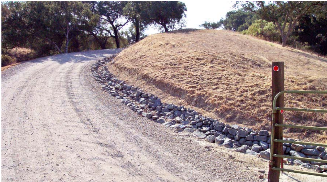
FIGURE 184. Rock armored ditches, if constructed with proper rock sizes, rock gradations and U-shaped channel form, can prevent ditch downcutting and erosion, but also inhibits easy ditch maintenance using machinery. Rather than armoring or installing check dams in ditches, it is usually best to reduce the volume of flow by installing additional ditch relief culverts.
