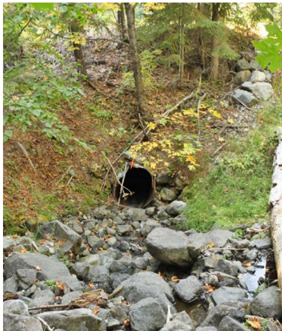
FIGURE 231. This 48-inch diameter culverted stream crossing in a steep, cobble and boulder bedded channel is dramatically undersized for the 100-year flow. The coarse bedload material and floating woody debris increase the potential for culvert plugging and overtopping of this large fill. Culverted stream crossings are considered the weak points of a road system. Not only can things go wrong easily, but the impacts of stream crossing failures are usually felt far downstream.
