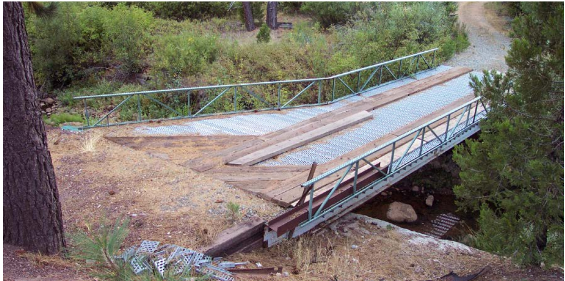
FIGURE 118A. This railroad flat-car bridge has been structurally modified to allow for some truck turning on the bridge deck. Deeply incised stream channels with steep sideslopes would require extensive hillslope excavation if a straight approach was utilized.
