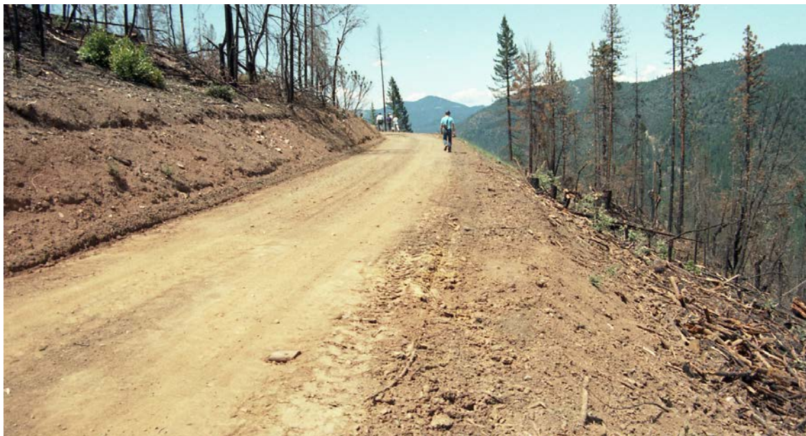
FIGURE 11. Seasonal roads are built to the same specifications as permanent roads, but are not surfaced for all-weather traffic. They typically provide summer or dry period access to watershed areas. The potentially erodible road surface may be waterbarred before each winter (not shown), or outsloped with rolling dips to provide for rapid drainage of surface runoff.
