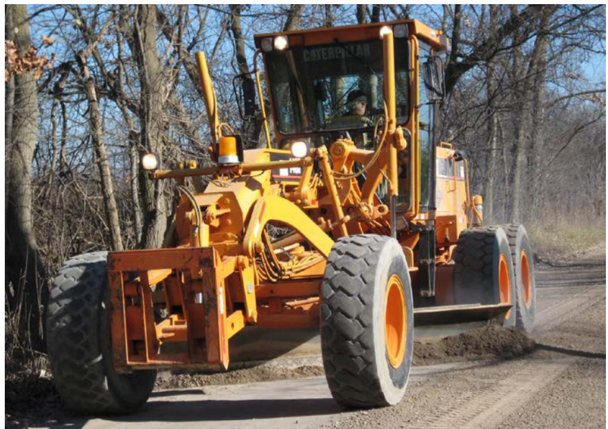
FIGURE 242. Grading a road to make a smooth running surface is beneficial for traffic, but it may also be treating the symptom of the problem rather than the cause of road roughness. Grading should have the dual purpose of 1) providing for a smooth running surface and 2) maintaining or improving road surface drainage. Grading for drainage will lower maintenance costs, as grading won't be needed as frequently. Grading only to produce a smooth road surface is a recipe for developing the exact same road problems that caused you to call for a grader.
