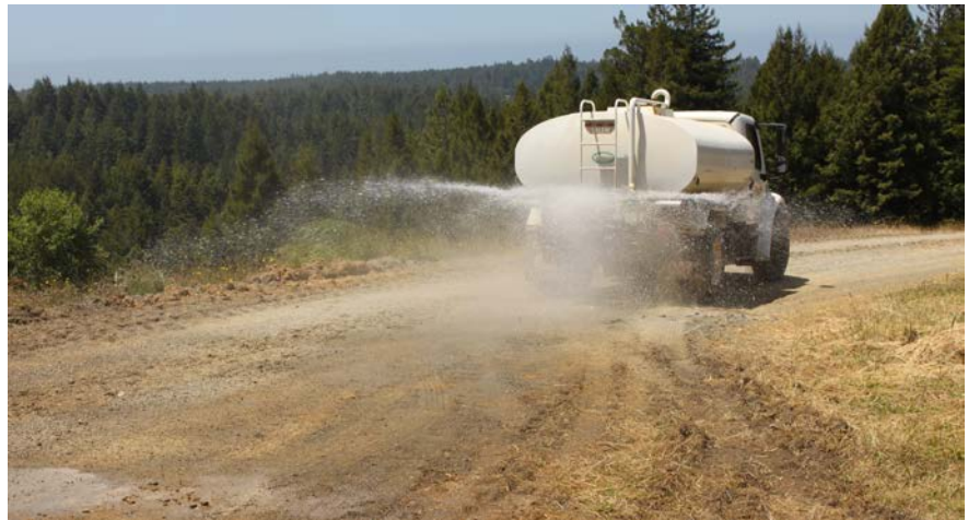
FIGURE 241. Water trucks can be used to apply water needed for compaction or dust control at project sites or along high traffic routes, or for applying a dust palliative (e.g., MgCl) for longer term dust control.
