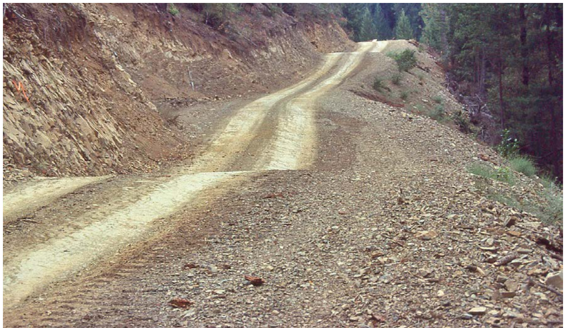
FIGURE 34. A classic Type I rolling dip, where the excavated up-road approach (B) to the rolling dip is several percent steeper than the approaching road and extends for 60 to 80 feet to the dip axis. The lower side of the structure reverses grade (A) over approximately 15 feet or more, and then falls down to rejoin the original road grade. The dip must be deep enough that it is not obliterated by normal grading, but not so deep that it is difficult to negotiate or a hazard to normal traffic. The outward cross-slope of the dip axis should be 3% to 5% greater than the up-road grade (B) so it will drain properly. The dip axis should be outsloped sufficiently to be self-cleaning, without triggering excessive downcutting or sediment deposition in the dip axis (Modified from: Best, 2013).
