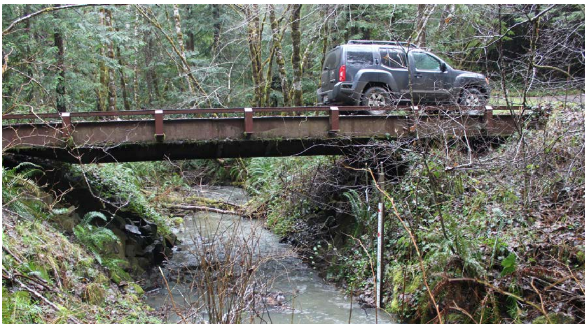
FIGURE 71. This 45-foot railroad flatcar bridge was installed to replace an undersized culvert that had been a barrier to fish migration. The channel width was maintained and a minor amount of armor was used to protect the abutments from erosion.
