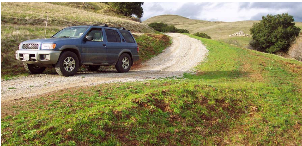
FIGURE 224B. The same road after being converted to an outsloped road with rolling dips to improve road drainage and decrease maintenance requirements and costs. The road was also gravel surfaced so it could be used during wet weather periods.
