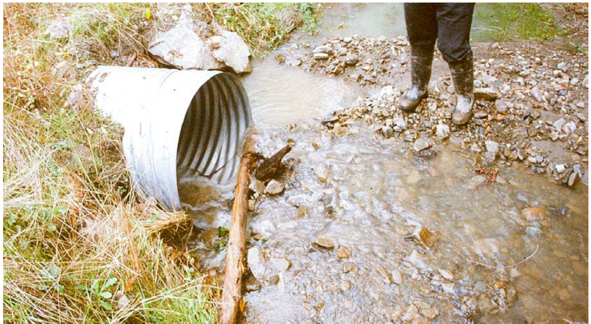
FIGURE 94. The inlet of this 30-inch diameter culvert shows considerable rust where bedload abrasion has worn away the galvanized coating and exposed the steel to corrosion (rusting). A rule-of-thumb for evaluating culvert sizing in the field is if the rust line in a galvanized steel culvert is higher than about 20% of the culvert diameter (i.e., active bedload transport is occurring high up in the culvert), then the culvert is probably undersized. This culvert displays a 50% rust line, suggesting it is very undersized.
