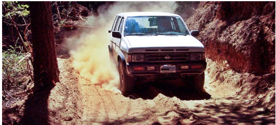
FIGURE 248 A & B. Excessive road dust during the summer (248a) and excessive mud during the winter (248b) are conditions which directly threaten water quality and result in high road maintenance costs. Both conditions produce and deliver large quantities of fine sediment to nearby streams during periods of surface runoff. This fine material can be especially damaging to fish and fish habitat.
