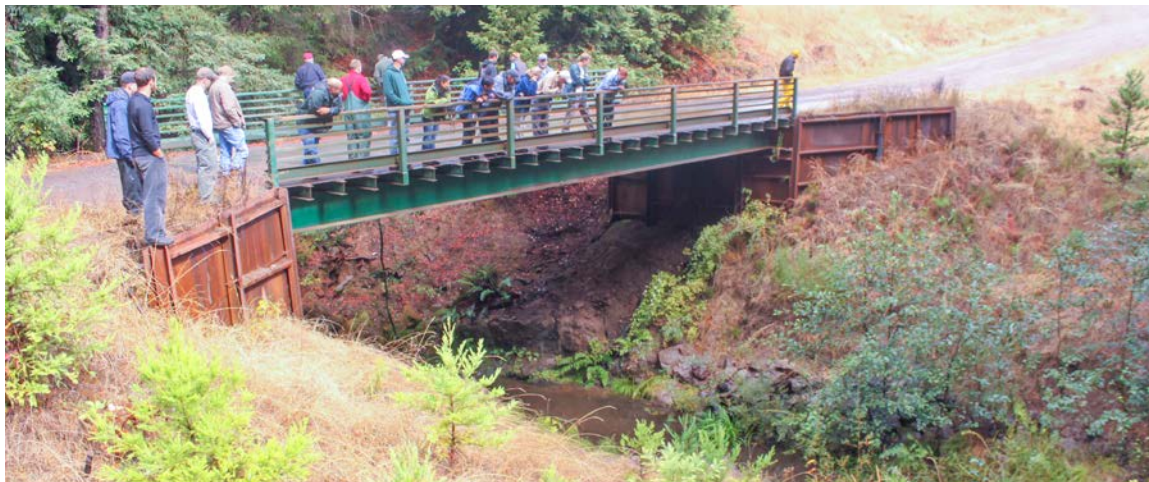
FIGURE 117. This 50-foot bridge is constructed from steel I-beams spanning the channel and secured to the slopes on either side of the channel using steel sheet pile abutments. I-beam bridges can be constructed on-site or they can be specified, prefabricated and assembled elsewhere, and then shipped and installed as a complete unit.
