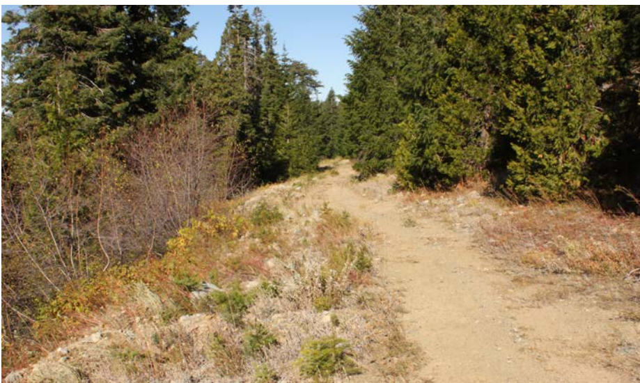
FIGURE 285. Former forest road that has been ripped, slightly out-sloped and converted to a hiking trail. The decommissioning treatment needed in this upper hillslope setting was minor and yet largely eliminated surface runoff from the alignment.
