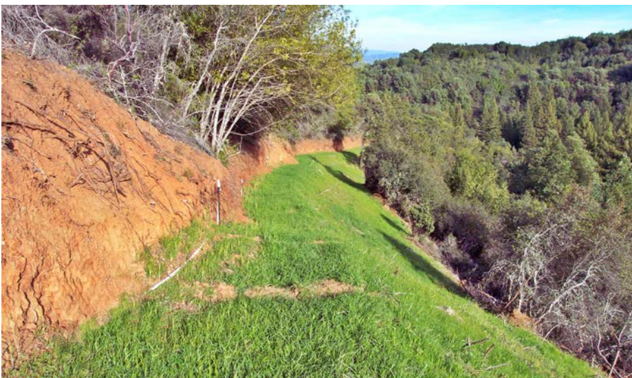
FIGURE 278. An illegally constructed road had been built across this steep hillside to access a new home site. Because of high erosion rates and slope instability, and because it was not permitted, regulatory agencies required the road to be fully decommissioned and recontoured. After excavation and recontouring, the bare slopes were seeded and watered to achieve a rapid and complete groundcover of grass. The decommissioning was approved to include a narrow trail for use as an emergency fire escape route, using small quads (off-road vehicles). A new and better alignment to reach the home site was subsequently found and constructed through proper permitting processes.
