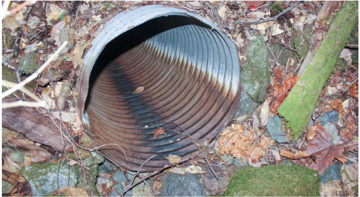
FIGURE 94. The inlet of this 30-inch diameter culvert shows considerable rust where bedload abrasion has worn away the galvanized coating and exposed the steel to corrosion (rusting). A rule-of-thumb for evaluating culvert sizing in the field is if the rust line in a galvanized steel culvert is higher than about 20% of the culvert diameter (i.e., active bedload transport is occurring high up in the culvert), then the culvert is probably undersized. This culvert displays a 50% rust line, suggesting it is very undersized.
