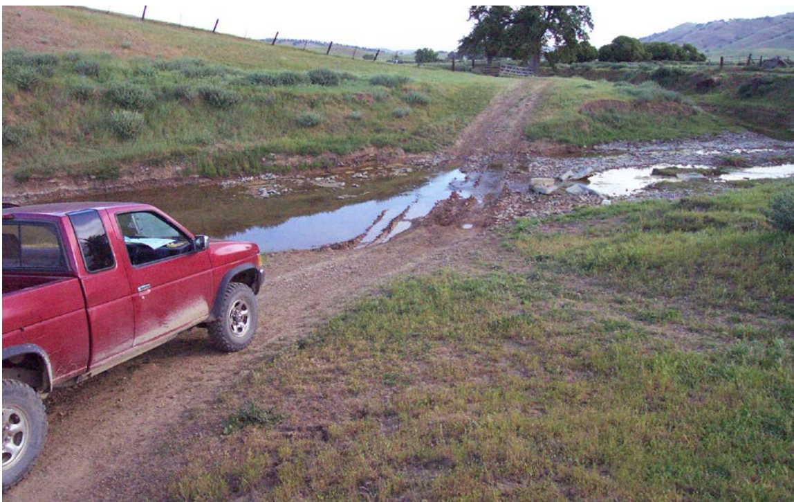
FIGURE 124. This unimproved ford crossing of an intermittent stream was poorly located in a channel reach that had a fine, erodible bed. Efforts to stabilize the channel bottom with rock and concrete chunks have been unsuccessful. A plume of turbidity is released in this fish bearing channel with each crossing.
