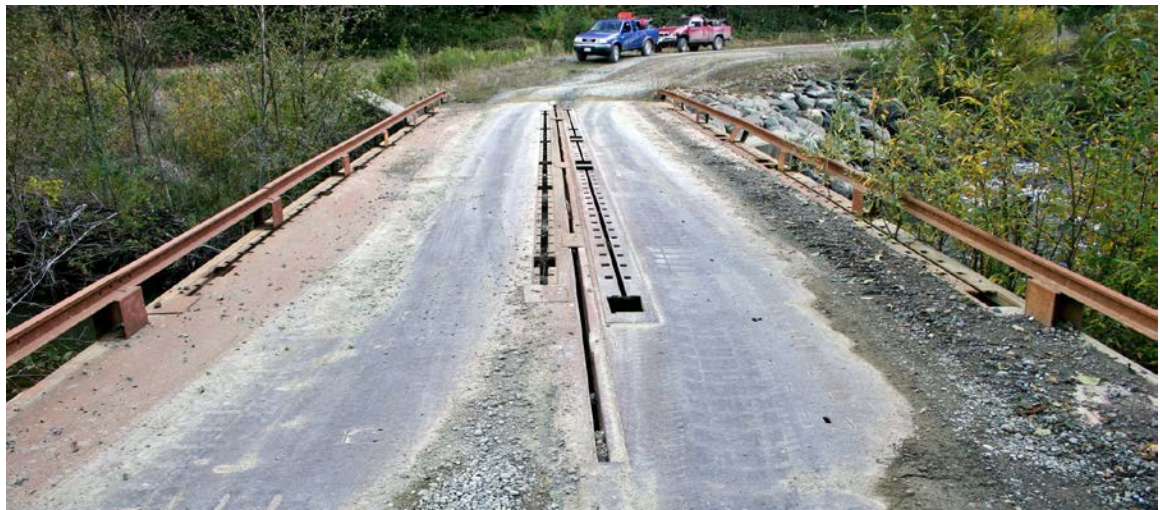
FIGURE 118B. Turning on the bridge can also be accomplished by using a double-wide flat-car bridge (two flat cars welded together), where the bridge width is sufficient to accommodate some turning by trucks with long trailers.
