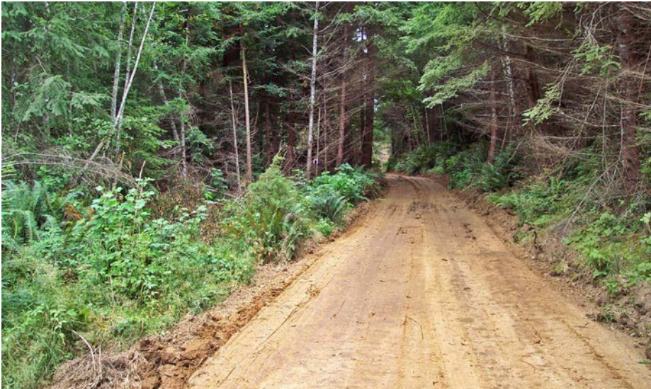
FIGURE 284A. On forest roads which are to be formally closed, rather than just “abandoned,” the roadbed can be returned to forest or grassland production by ripping and disaggregating the surface and then planting with trees. Figures 278a and 278b show a road before and after ripping and decompaction. This simple, inexpensive treatment also helps reduce runoff from compacted areas. It is recommended that enough passes be made with the tractor so the surface is completely disaggregated.
