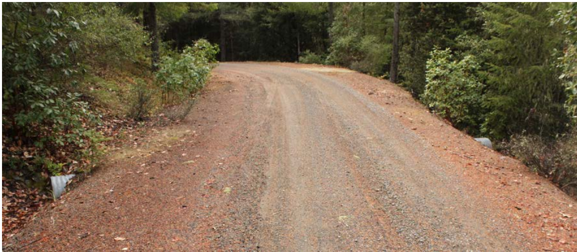
FIGURE 48. The elements of a properly installed ditch relief culvert. The culvert is angled at about 30 degrees to the road alignment to help capture flow and prevent culvert plugging or erosion of the inlet area. It is set at the base of the fill (ideally) or with a grade slightly steeper than the grade of the contributing ditch (but never with a grade less than 2 percent). At a minimum, the grade of the ditch relief culvert should be sufficient to prevent sediment accumulation at the inlet or deposition within the culvert itself (it should be self-cleaning) (USDA-SCS, 1983).
