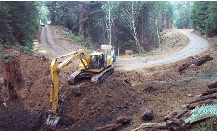
FIGURE 266B. Once cleared, an excavator excavated the fill material and several dump trucks were used to end-haul spoil material to a nearby, stable disposal site.
