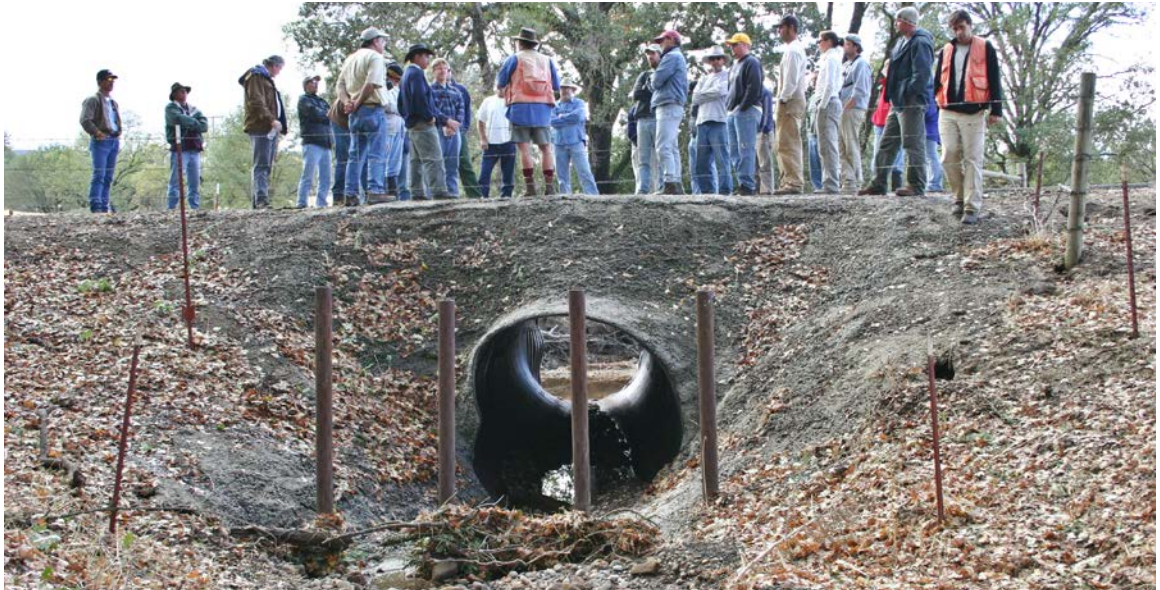
FIGURE 104. The most effective trash rack or screen is one placed across the channel slightly upstream of the culvert inlet, with the spacing of the vertical posts approximately equal to the span or diameter of the culvert. Closer post spacing catches too much debris, and wider spacing lets large debris through that could plug the culvert inlet. The 4 posts on this debris rack are a little too closely spaced and one more post should be added to each side to prevent flanking during a flood event.
