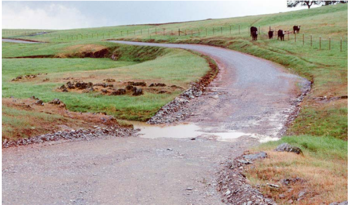
FIGURE 125. In addition to the actual ford crossing, the road approaches also contribute to sediment pollution unless they are paved or heavily rock surfaced. Fords are always low points in the road, so runoff from the connected approaches is delivered directly to the stream channel.
