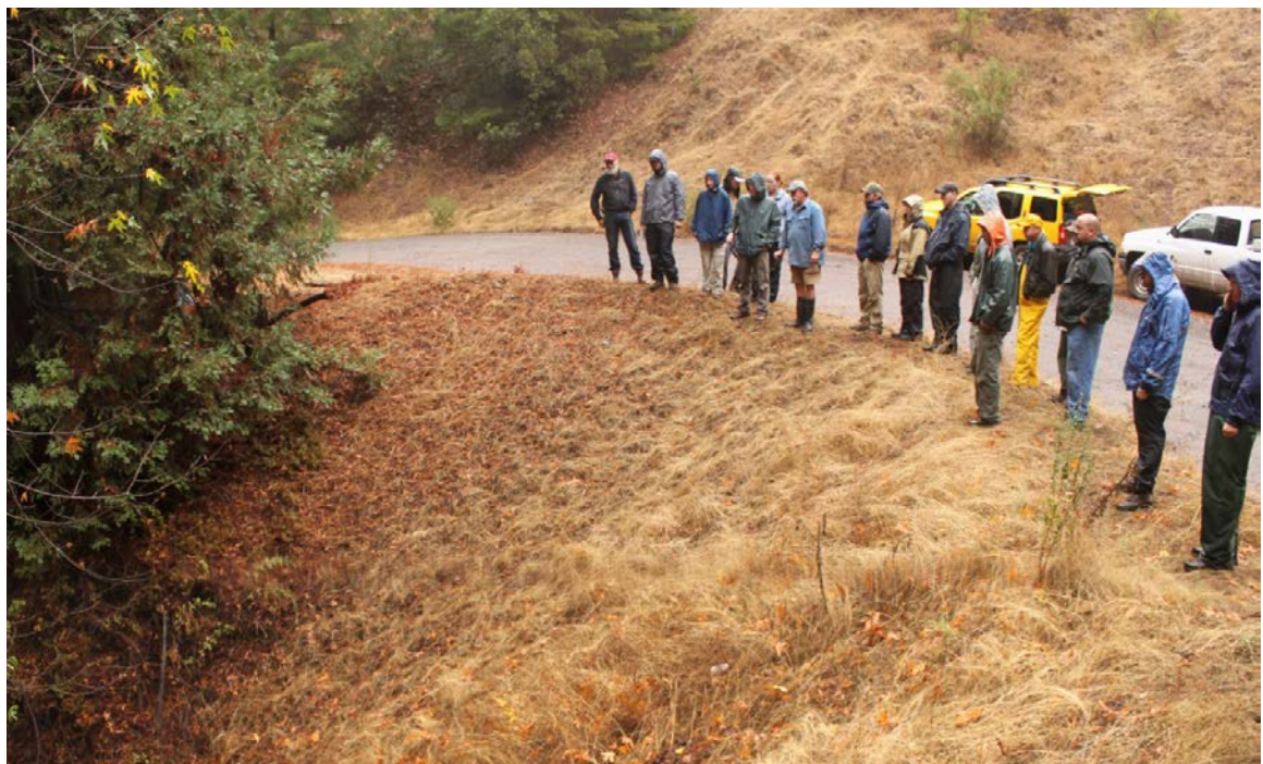
FIGURE 175. Mulching and seeding are effective methods for controlling surface erosion from bare fill slopes. Mulch protects the soil until the grass and vegetation is firmly established. However, because it decomposes rapidly, straw mulch is effective for only the first year. After that, well established vegetation should provide the needed protection.
