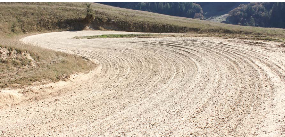
FIGURE 167. Dry rock dust is formed by heavy traffic or commercial vehicles mechanically abrading and wearing down road surfacing materials. The road surface wears down and sediment leaves the road as airborne dust or in runoff during the next runoff event.
