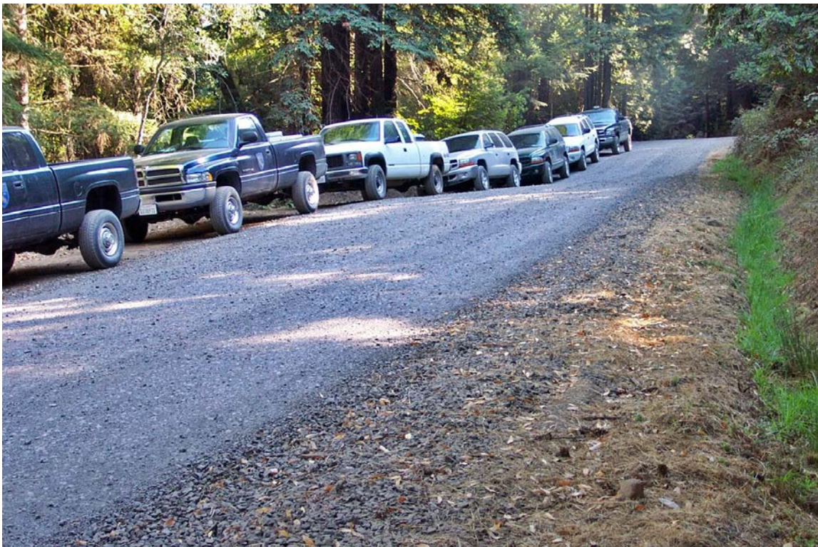
FIGURE 43. This rural subdivision road has been converted from an insloped, ditched road to an outsloped road shape with rolling dips and an inside ditch. Broad rolling dips have been built at regular intervals to accommodate all traffic types. The ditch has been retained to drain clear spring flow from the small cutbank. The road surface no longer drains to the ditch.
