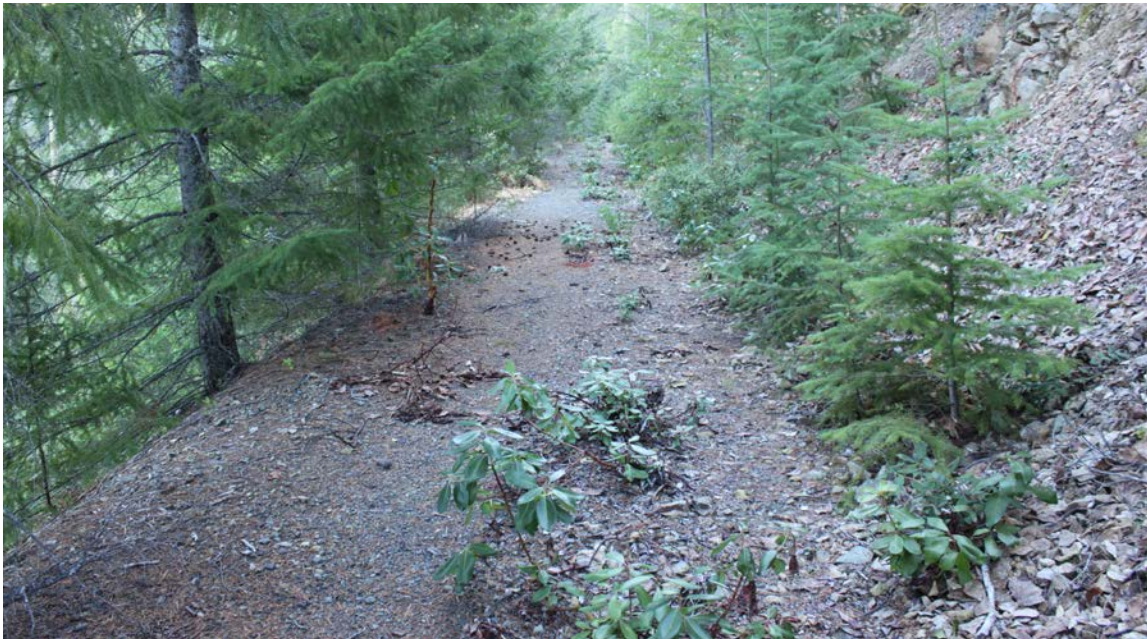
FIGURE 260. Untreated, abandoned section of forest road does not threaten water quality and needs little or no treatment for decommissioning. Roads to be decommissioned typically require minimal treatment for most of their lengths, and then concentrated erosion prevention work at a relatively few locations (e.g., stream crossings).
