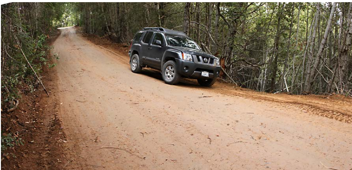
FIGURE 164. On steep roads (over about 15% to 18%) reverse grade rolling dips are short and steep, and may be difficult for some traffic to pass. Alternately, a Type 3 rolling dip can be constructed where road surface runoff is drained off the road by locally increasing the outslope rather than reversing the grade with a dip. (See Figure 36).
