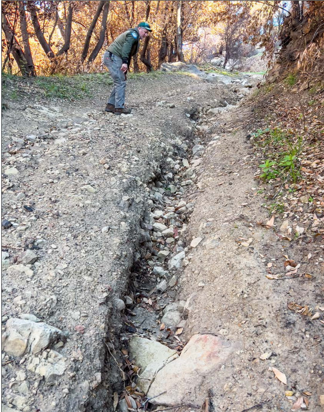
Gullied section the Restoration Management Plan proposed language would not allow cutting into the outside berm to create a more sustainable trail.
